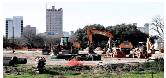
Elm Avenue construction - June 2020
