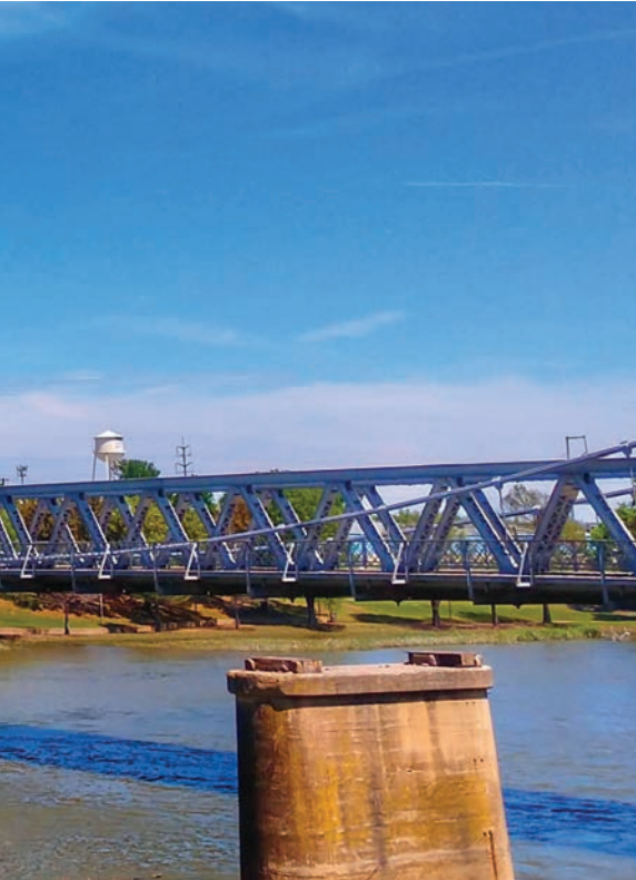
Waco Suspension Bridge June 2020
