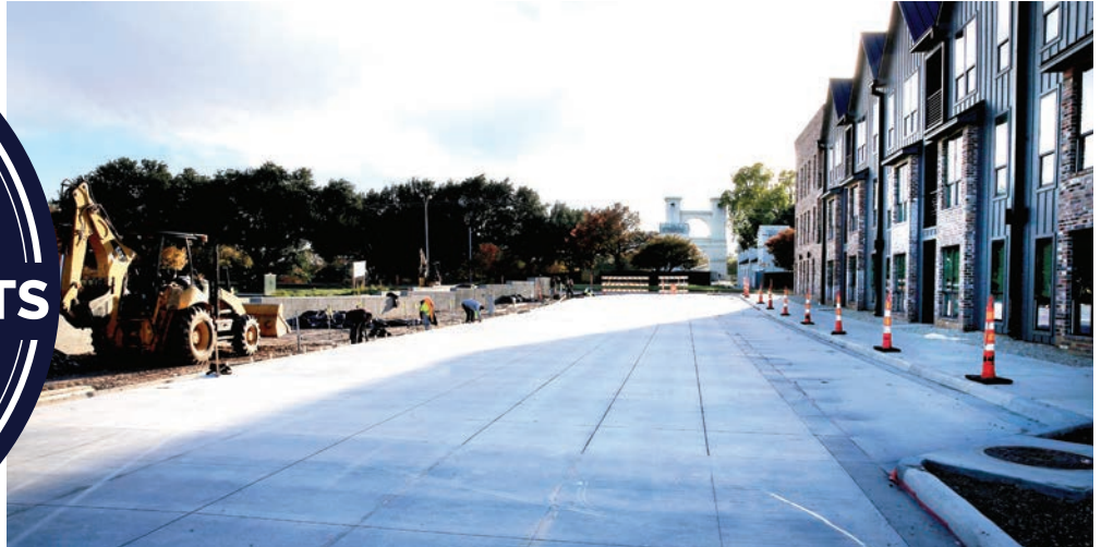
Bridge Street construction - December 2020
