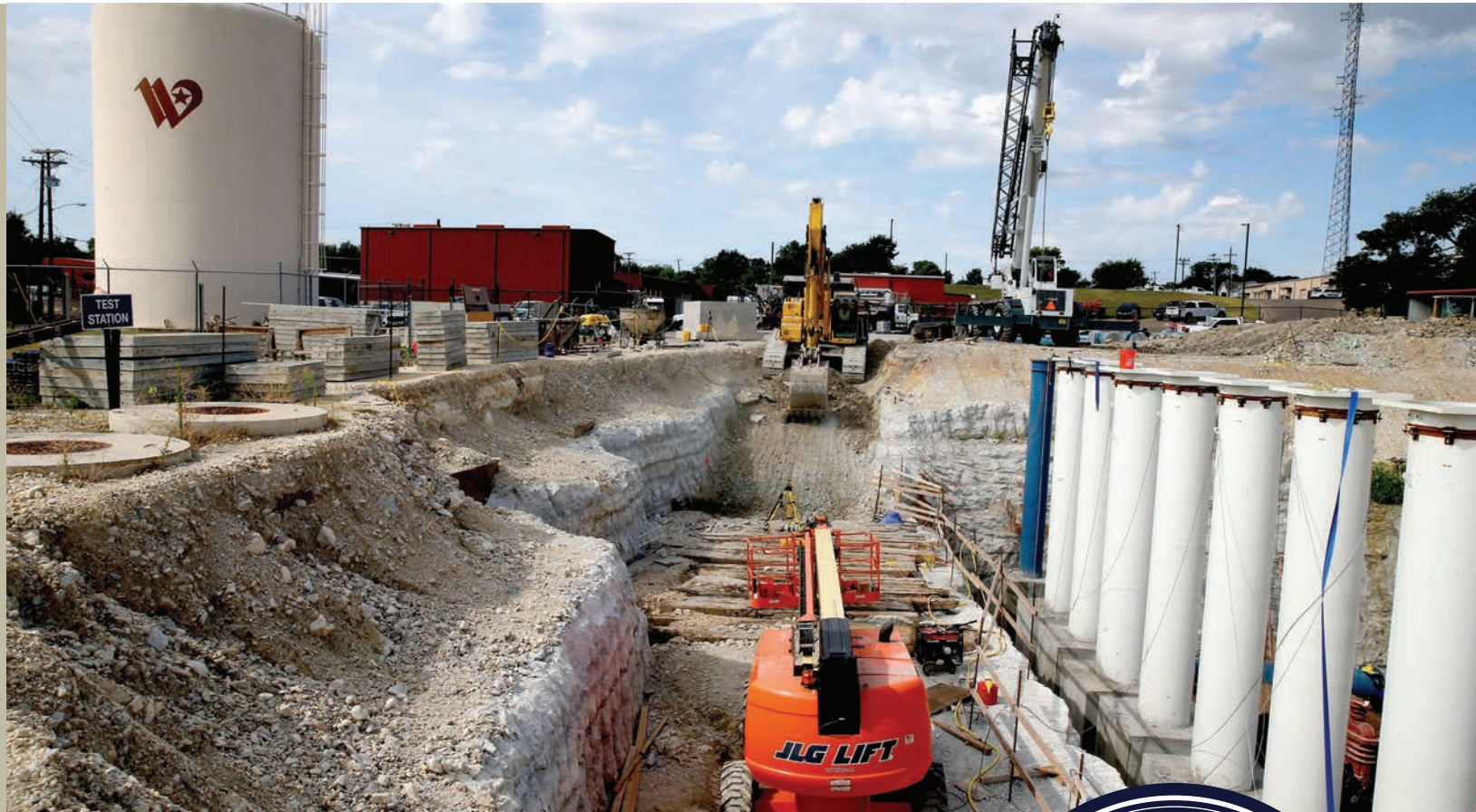
Riverside Treatment Plant Pump Station Construction - July 2020
