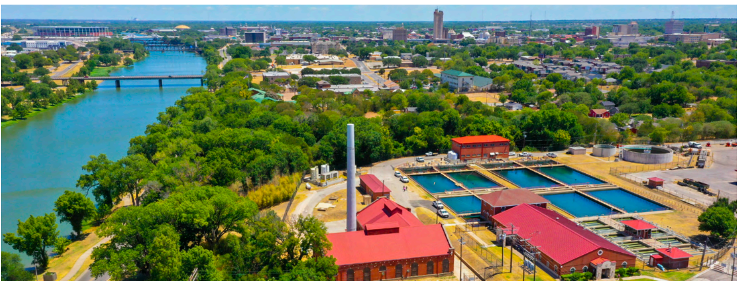
Riverside Water Treatment Plant.
