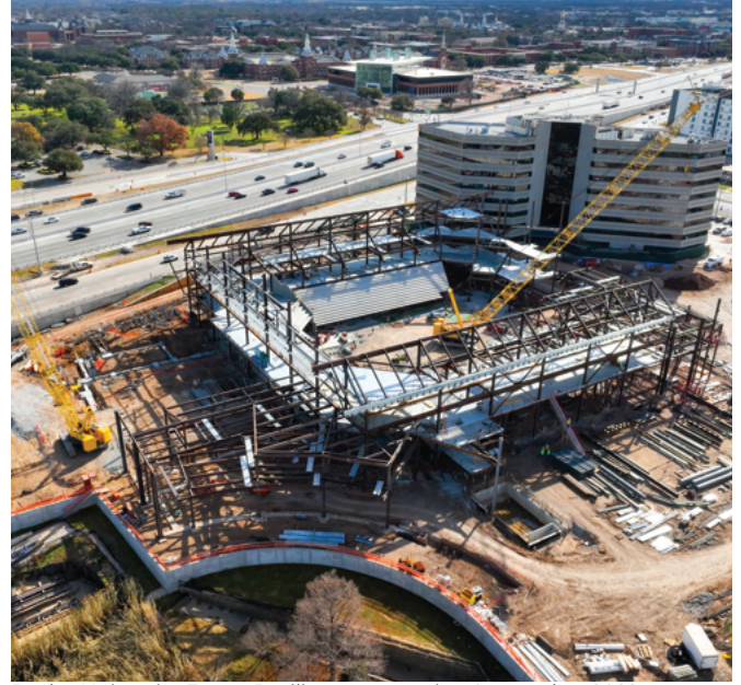
Baylor University Foster Pavilion construction September 2022.
