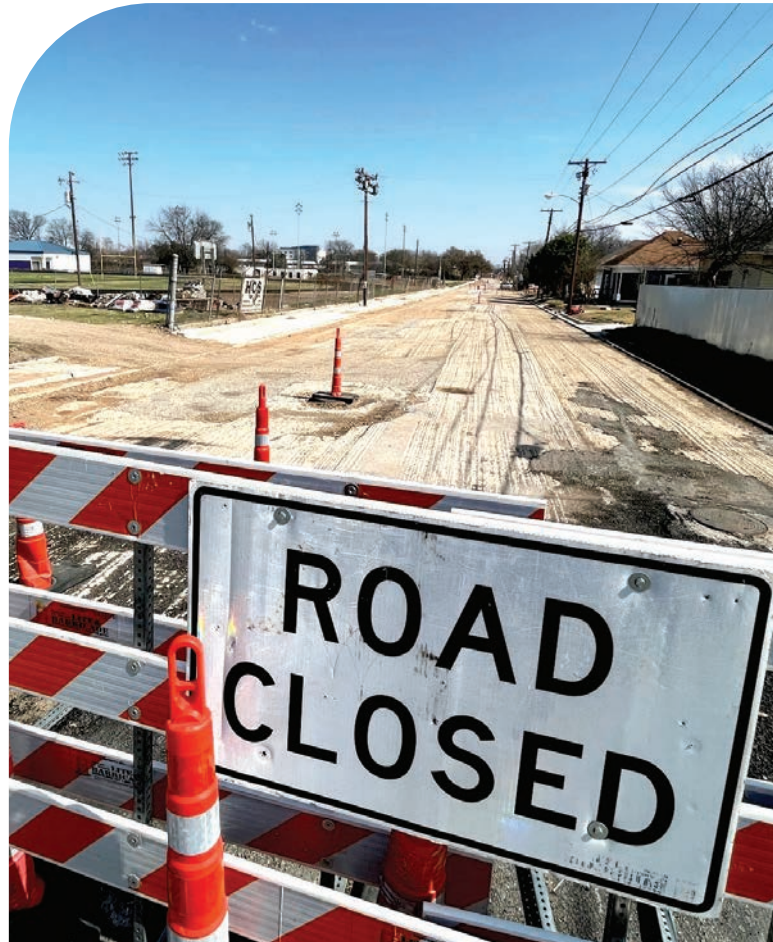
Construction continues on Dutton Avenue - December 2021.
