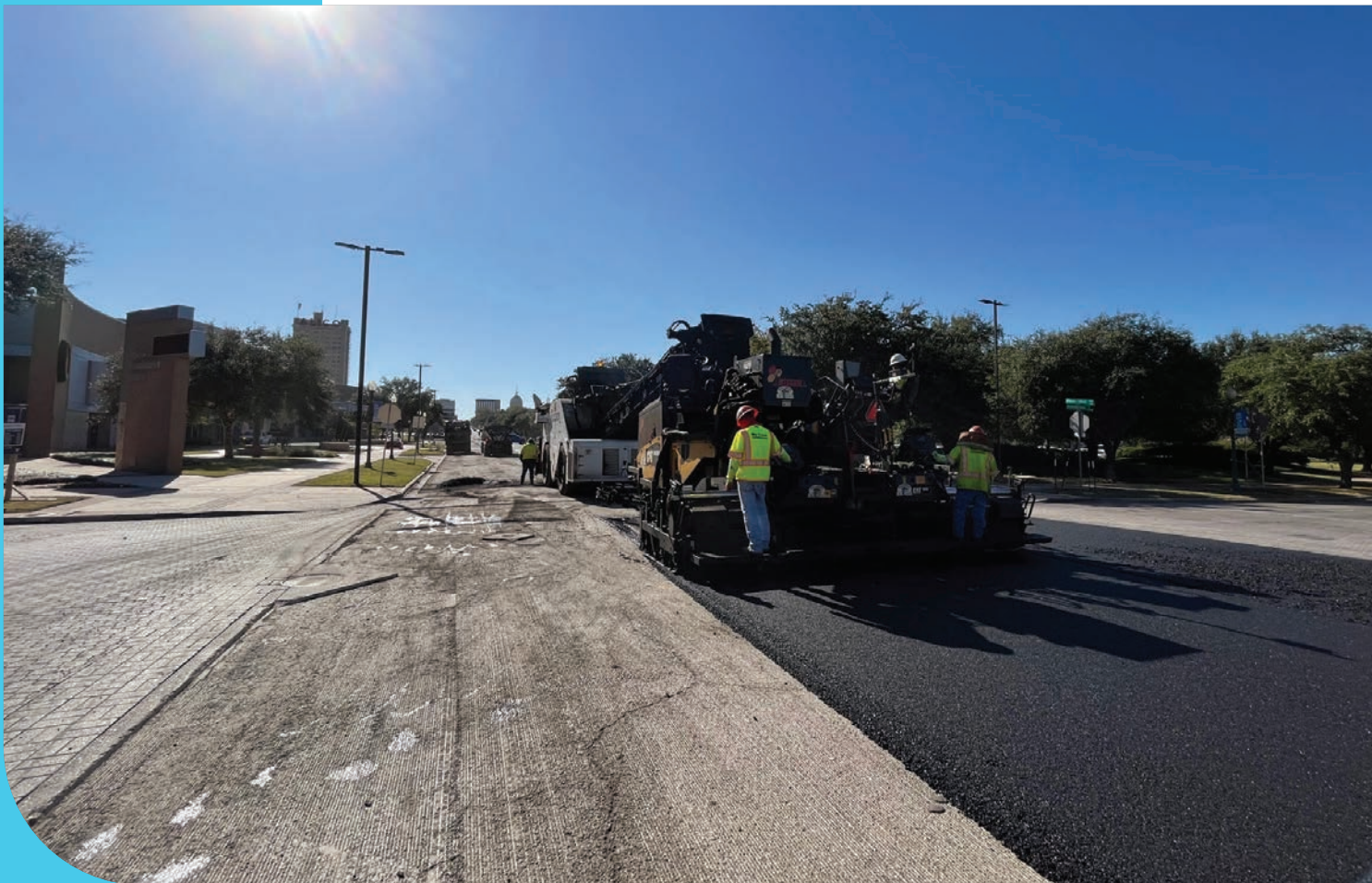
Paving Washington Avenue in Downtown Waco - November 2021.
