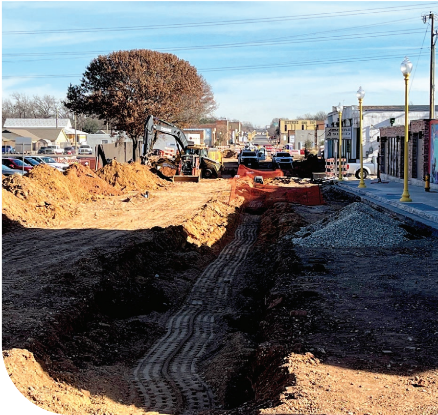
East Waco, Elm Avenue Construction - October 2021.
