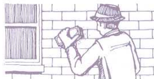
Bristle brushes are recommended over metal brushes since metal can damage the mortar and masonry.
